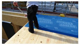
6. Rub the membrane firmly to secure the adhesive bond
