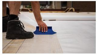
4.2 Install the membranes, making use of the release film splits
