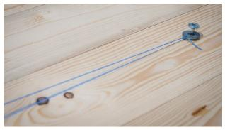
**3.1 Create marking** Mark the position of the first membrane on the subsurface.
