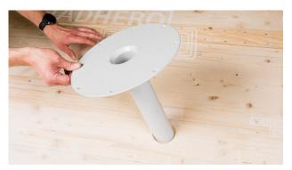
9. Drainage: Installation of ADHERO Floor Drain Insert the ADHERO Floor Drain into the drillhole and, if necessary, secure with countersunk screws.
