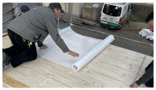
4.1 Install the membranes, making use of the release film splits
